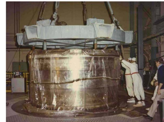
Handling of Upper Concrete Plug
