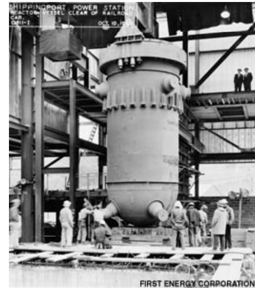
Shippingport Pressure Vessel Operational – 1957 (60 megawatt-electric)
